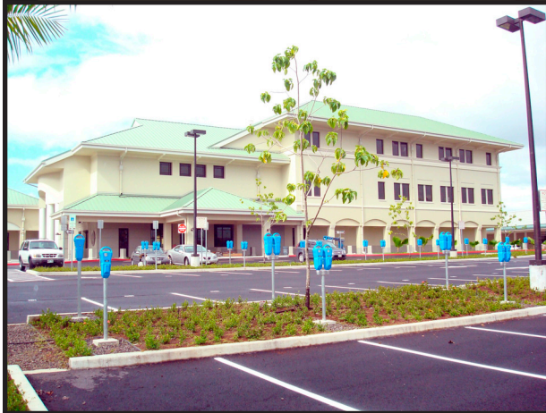
Photos above: The Hilo Judiciary Complex, named “Hale Kaulike” (House of Justice), was opened to the public on March 30, 2009.
